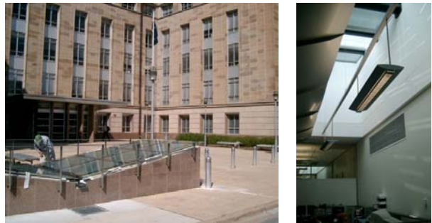
Figure 6. External and internal views of skylight penetrations.
