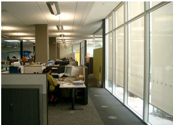
Figure 5. Suspended luminaires, and external screens on courtyard windows.
