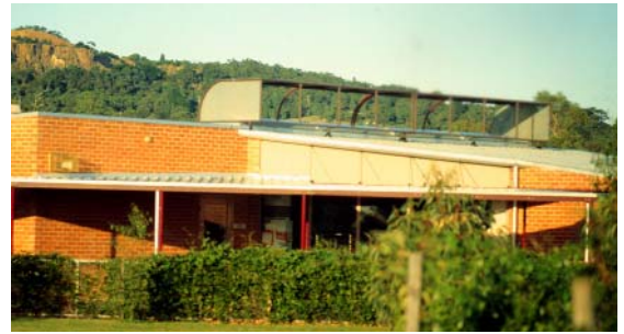
View from northeast, showing skylight and window shading.
