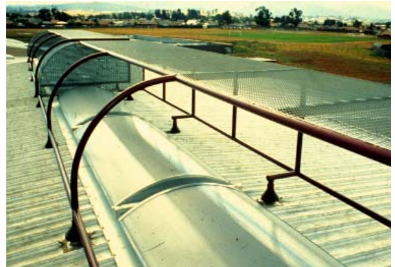
External view of skylight with steel mesh shading.
